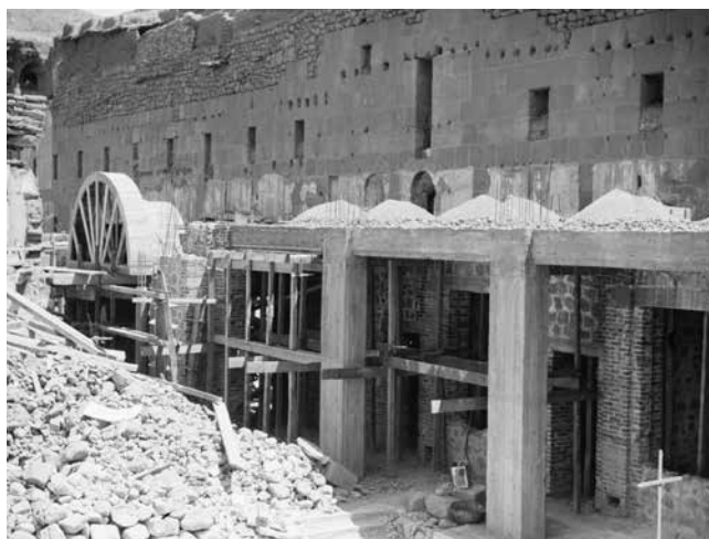
5. Construction of the ground floor, South Range (Matson Collection, 1933).
