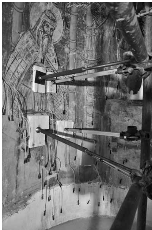
Chapel of the Prophets Moses and Aaron: preparation for grouting.
